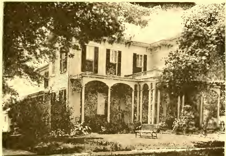
RESIDENCE OF GORTON D. JERAULD. Corner South and 6th Streets.
